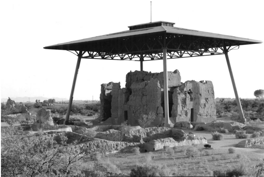
Fig. 2. Great House at Casa Grande under modern protective roof (Photo courtesy of the United States National Park Service).
